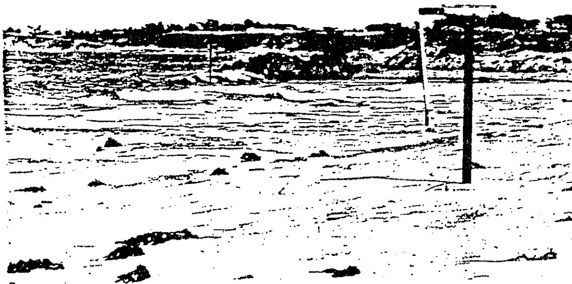
Fig. 5.- Freshwater pipes now in the sea. East end of the basalt wall and continued erosion in foreground.
