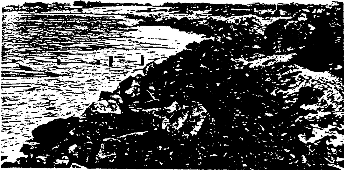
Fig. 3.- The basalt wall placed on the back beach to halt erosion. The sea removed the sand on the seaward side of the wall, admitting the waves further inshore, and so facilitating back-wall erosion. The wall was raised in 1963 and in 1979 is being further raised. Loss of a beach seaward of a seawall is the usual result. I am informed that the stumps in the photo are of an experimental groyne
