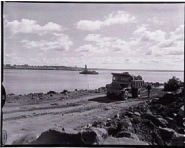
Figure 10 - Construction of the new breakwater (SLV: Victorian Railways 1955 Accession No: H91.330/4283)
