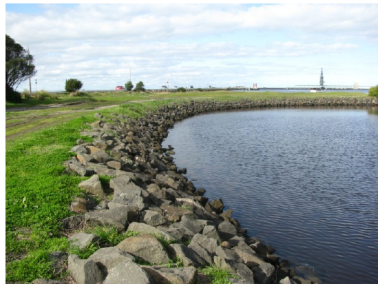
Plate 2 - Sea-wall protecting reclaimed area
