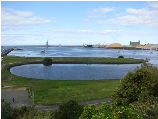
Plate 1 - Reclaimed area next to breakwater
